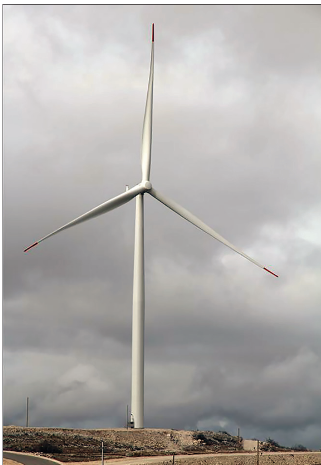
Figure 2.35 WF Mesihovina, 50.6 MW, in operation since 2018
