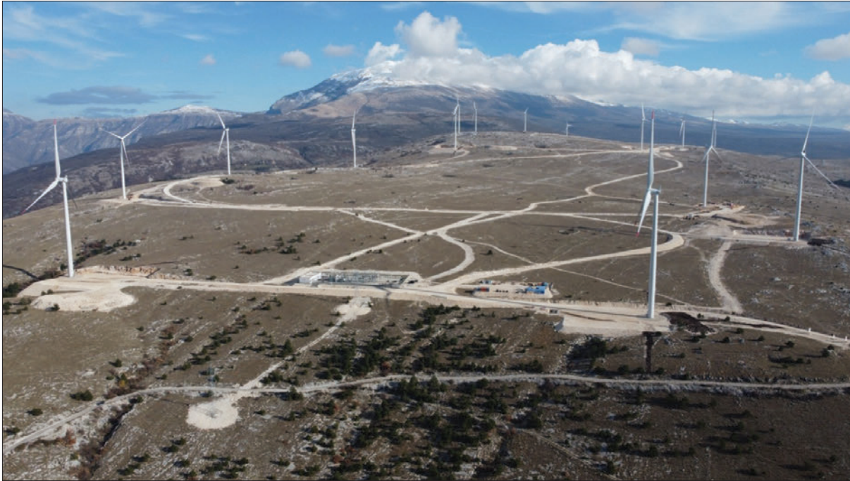
Figure 2.37 WF Podveležje, 48 MW in operation since 2021
