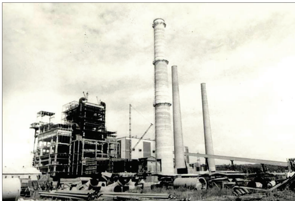
Figure 2.24 TPP Tuzla, III stage, 1971
