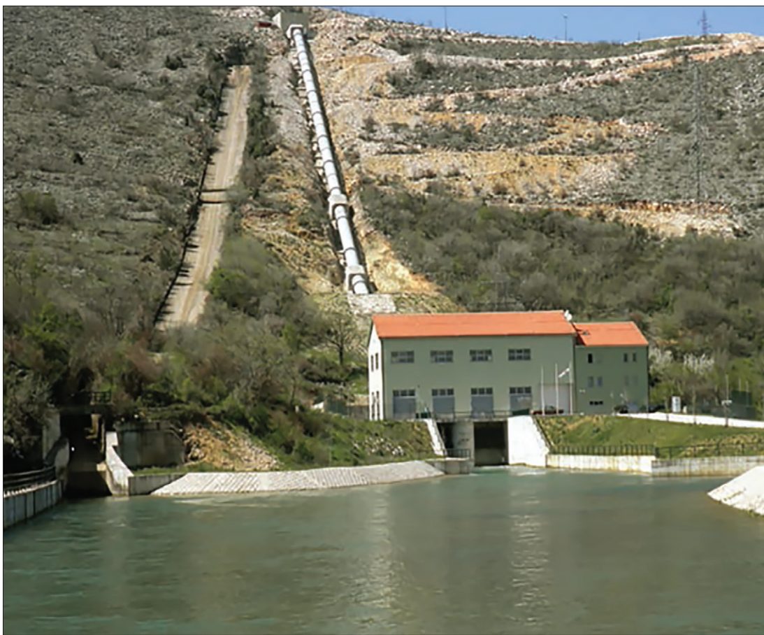
Figure 2.33 HPP Mostarsko blato, 60 MW, in operation since 2010
