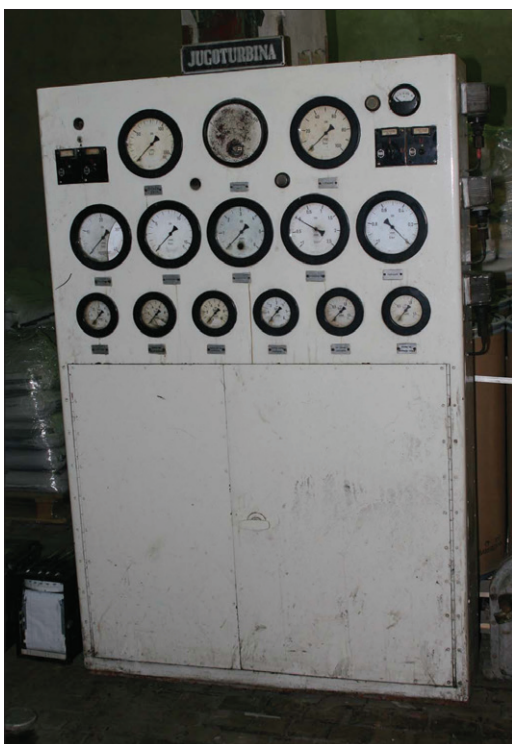
Figure 13.10 Instrument panel in front of the turbine for monitoring the operation of the 32 MW turbine (production 1956)
