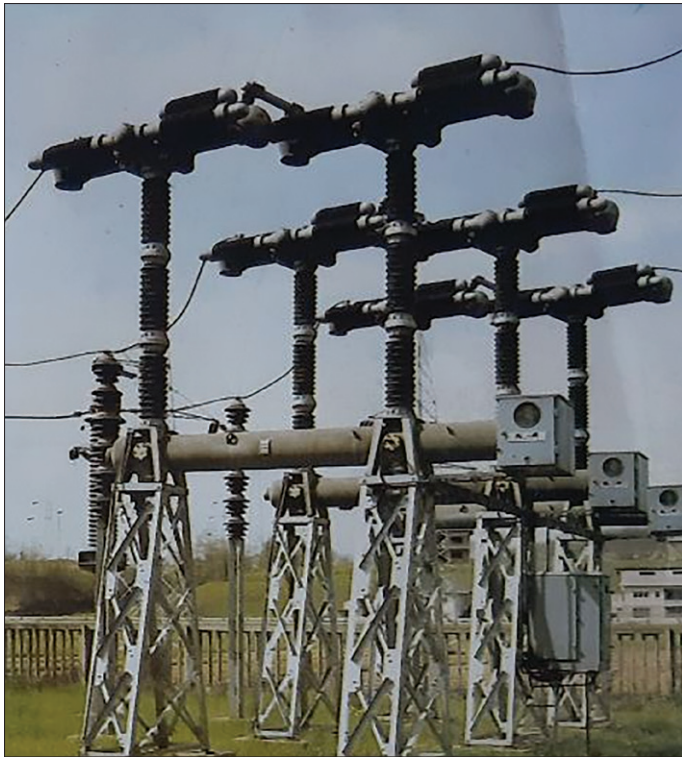
Figure 3.14 Energoinvest's high-power laboratory, a) protection breaker, 1985
