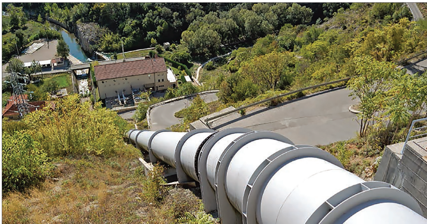
Figure 2.32 HPP Peć Mlini, 30.6 MW, in operation since 2004
