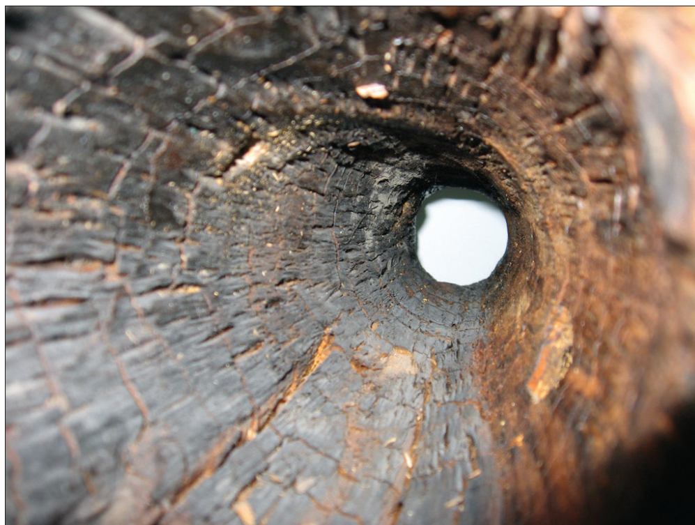
Figure 13.17 “Tomruci” interior of a wooden water pipe
