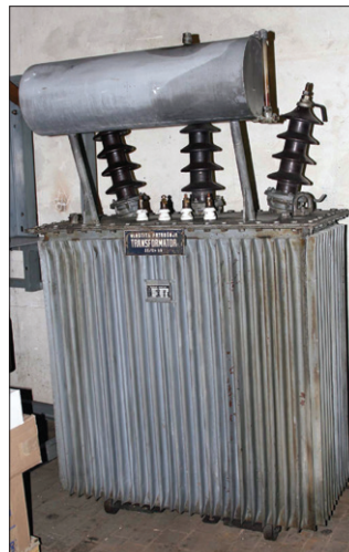
Figure 13.13 Transformer 35/04 kV (produced in 1956 by RADE KONČAR)
